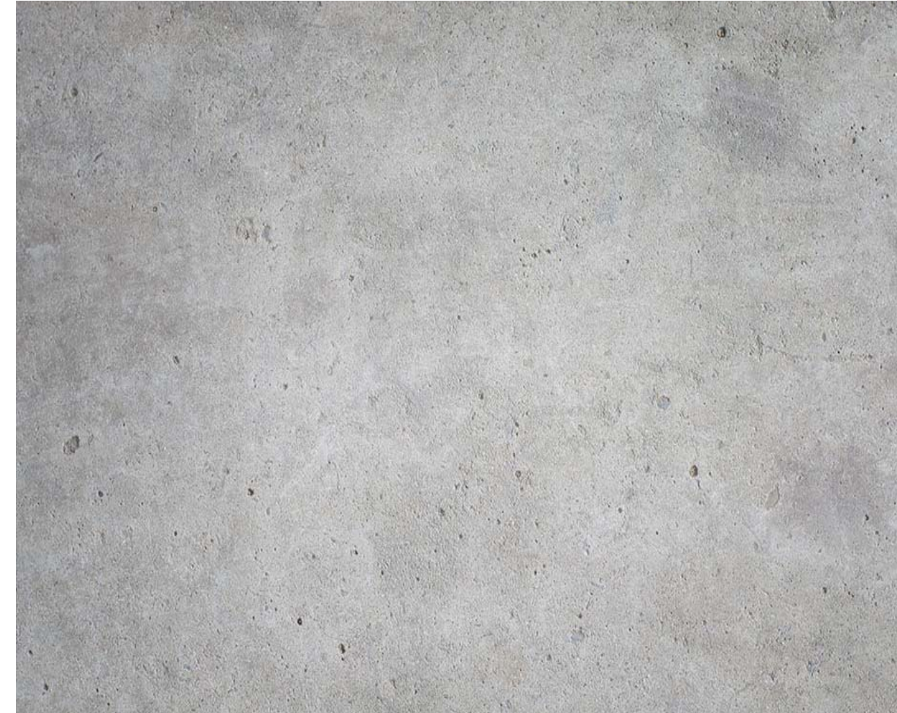
8 EXPOSED ARCHITECTUAL CONCRETE
