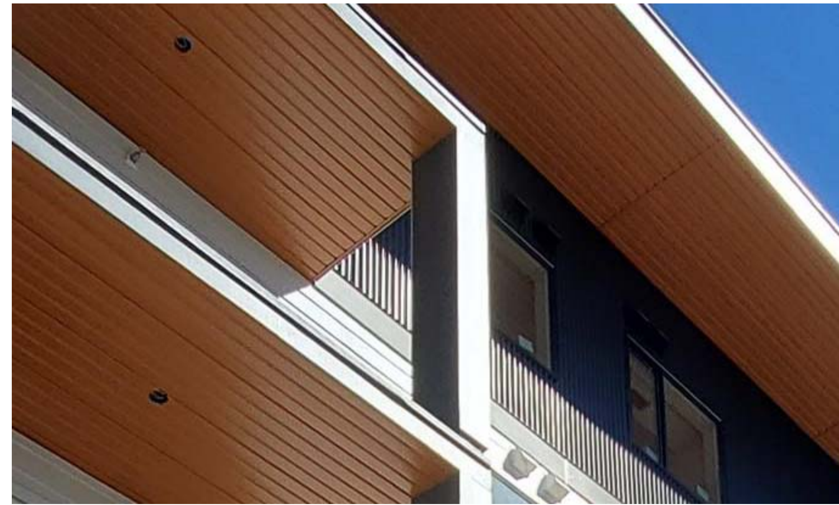
4 PRE-FINISHED ALUMINUM SOFFIT COLOUR: 527 - CEDAR XL MANUF/STYLE: GENTEK 2345 VENTED SOFFIT
